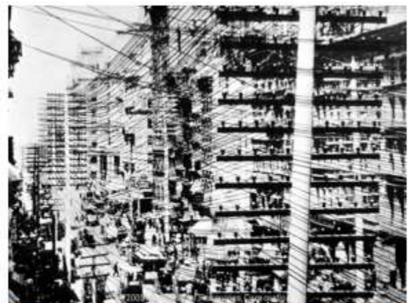
New technologies grew quickly in the 1880s. Telephone and electric wires, like the ones on this New York City street in 1884, brought new services to consumers.
